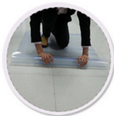
5、 Roll the mat from the oppsite site
