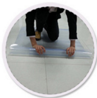
5、 Roll the mat from the oppsite site
